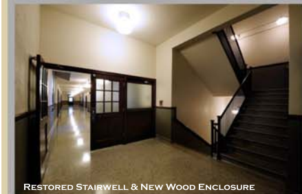
RESTORED STAIRWELL & NEW WOOD ENCLOSURE
